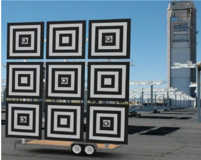
Figure 73. Target used for TOP alignment technique on heliostats.
