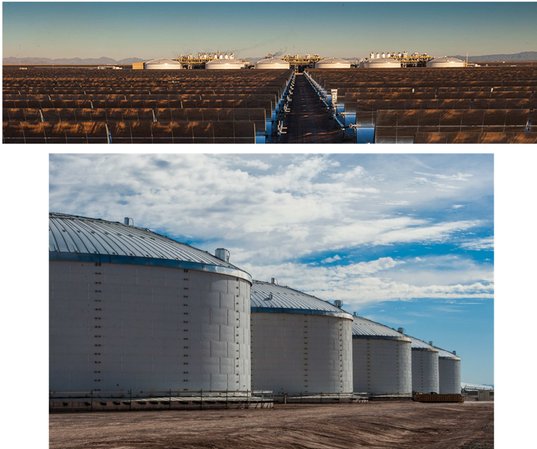
Figure 12. Solana solar thermal power plant with two-tank molten salt storage system (source: Abengoa)
