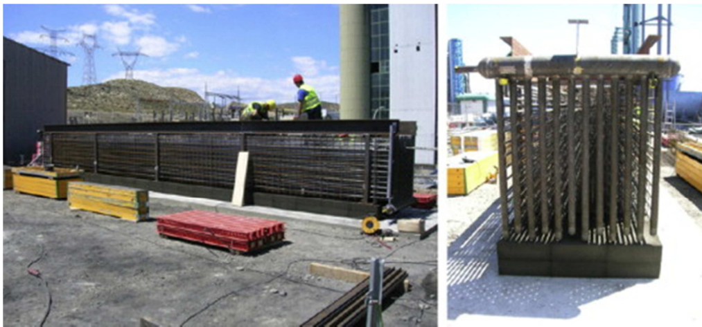
Figure 14. Prefabricated tube registers being installed in a concrete storage test module at DLR [Laing 2011].
