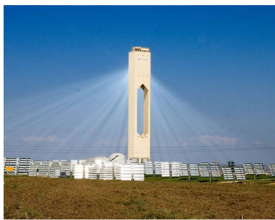
Figure 6: 11 MW e saturated steam PS-10 plant in Seville, Spain.
