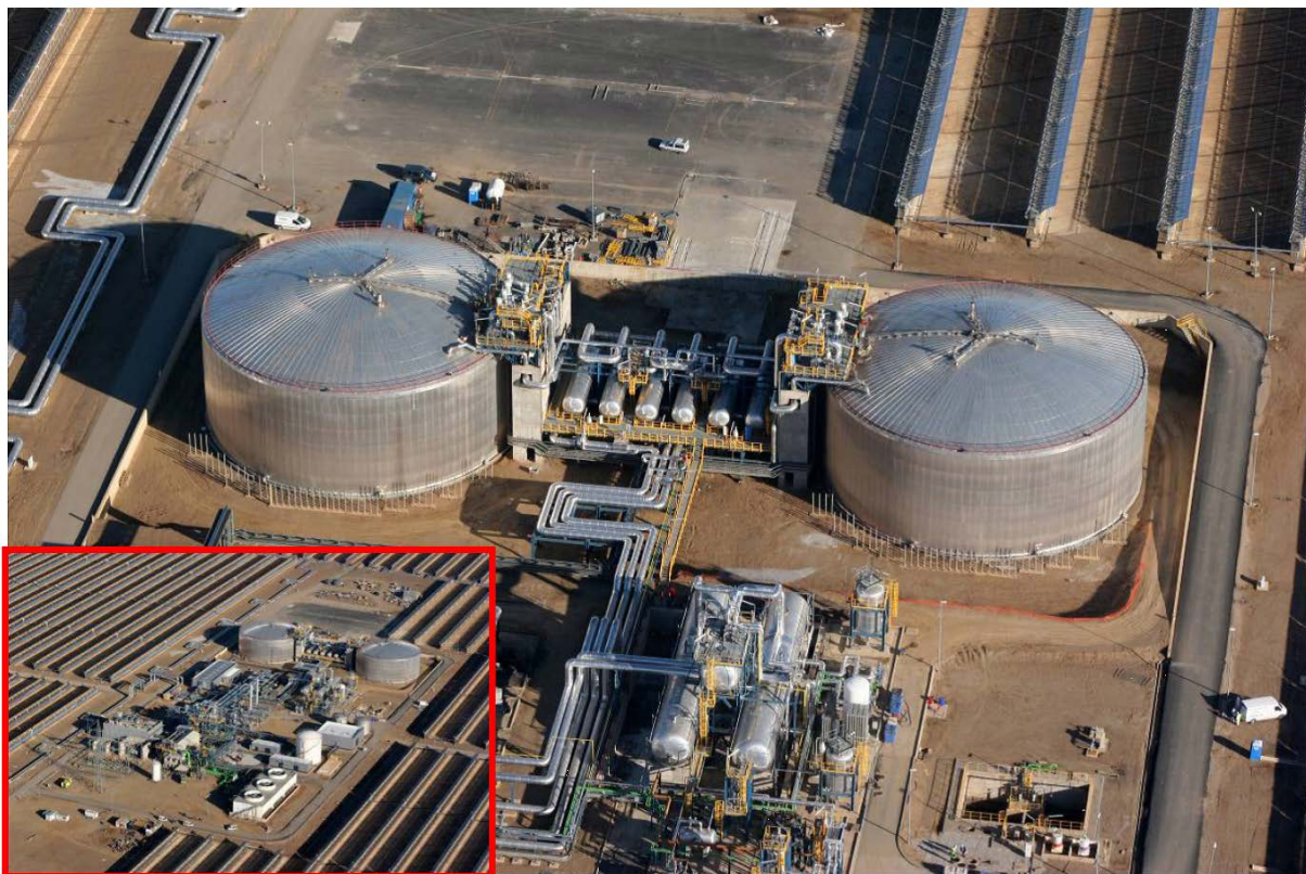
Figure 10: Aerial view of the Andasol plant in Guadix, Spain, showing the power island (insert) and details of molten-salt storage tanks and heat exchangers.
